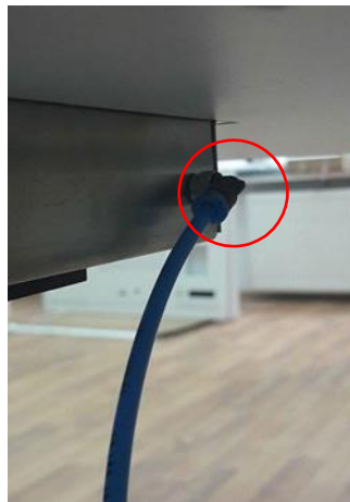
Figure 34.9 Gas line connection under the tabletop
